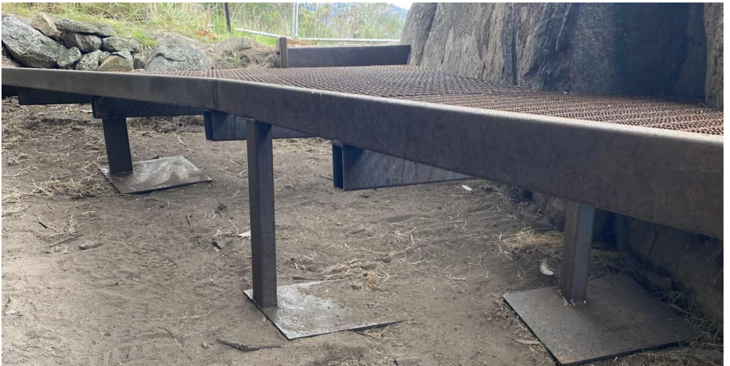
Steel plates support the new viewing platform so that it stands free of the rock and leaves the soil free of disturbance.
