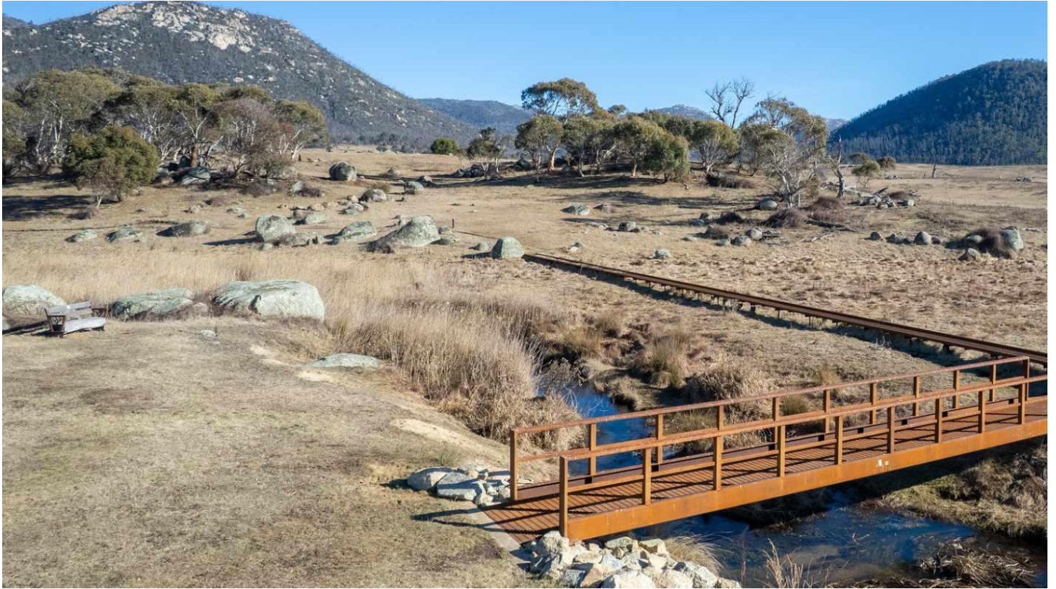
The stone and steel fabric of the new footbridge and boardwalks will better withstand future fires.
