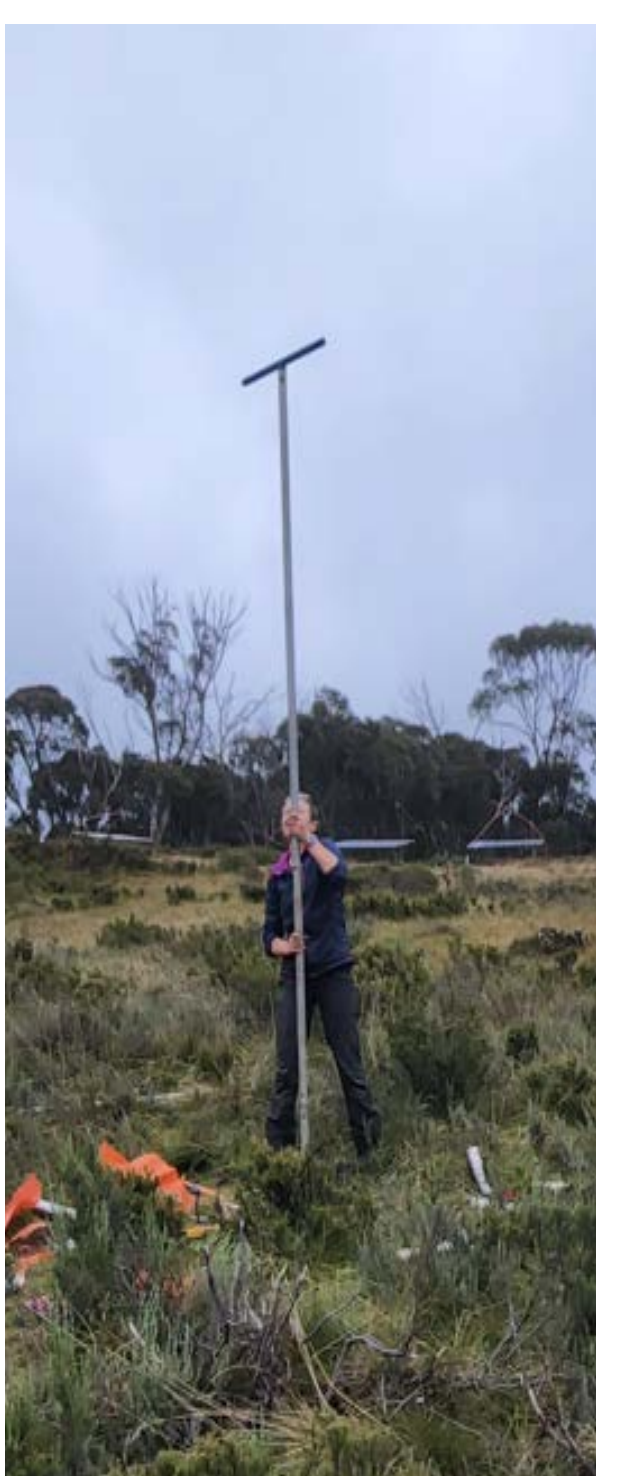
Borehole Piezometer Installation at Perisher
