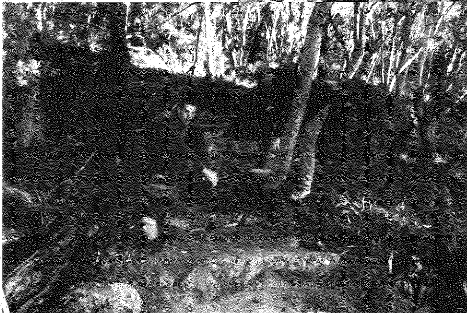
Above Hardwood Steps and water diversion bars sourced from a powerline clearing activity.
