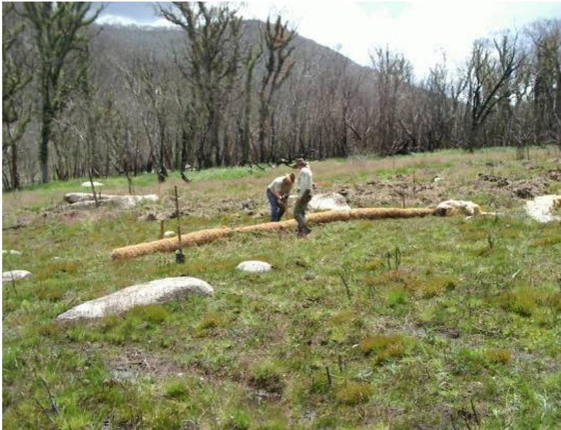
Figure 3. Coir logs placed on the contour to prevent flow-line formation and to act as water-spreaders of surface runoff into bogs and fens.
