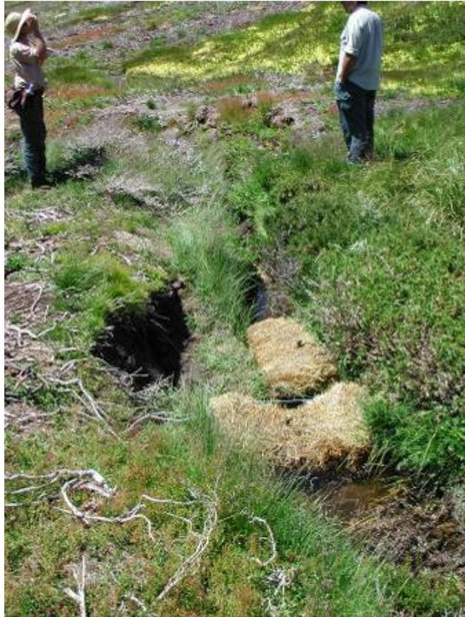
Figure 6. Three or four layers of straw bales packed into an incised flowline to prevent lateral undercutting and peat collapse.
