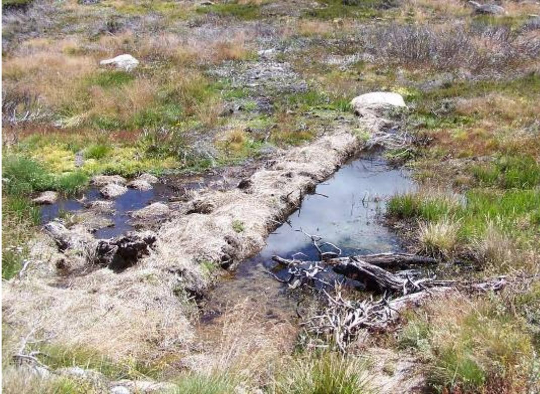
Figure 8. One hundred metre long subsurface ‘straw-bale dam’ (partly exposed for demonstration) to assist the retention of inflows in the peat during resaturation.
